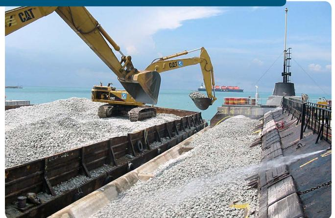
However if the outreach of the excavator is limited, there is an inherent possibility that the dredged material will drift and re-enter the excavated area. Loading excavated material into barges for transport remains the most common means of disposal.
