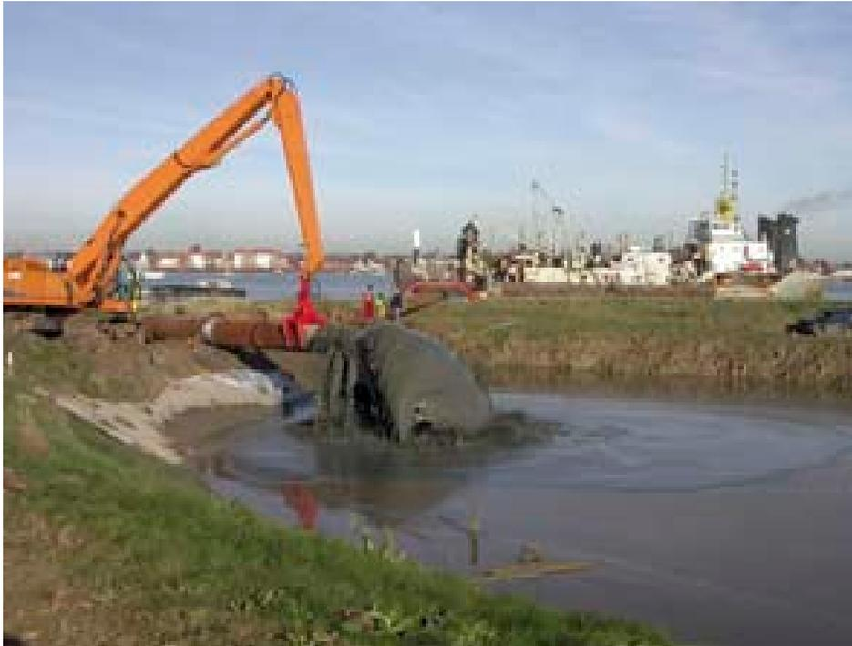
Figure 4. The dredged material was pumped through a pipeline from the vessel into a containment bund on the seaward side of the new seawall.
