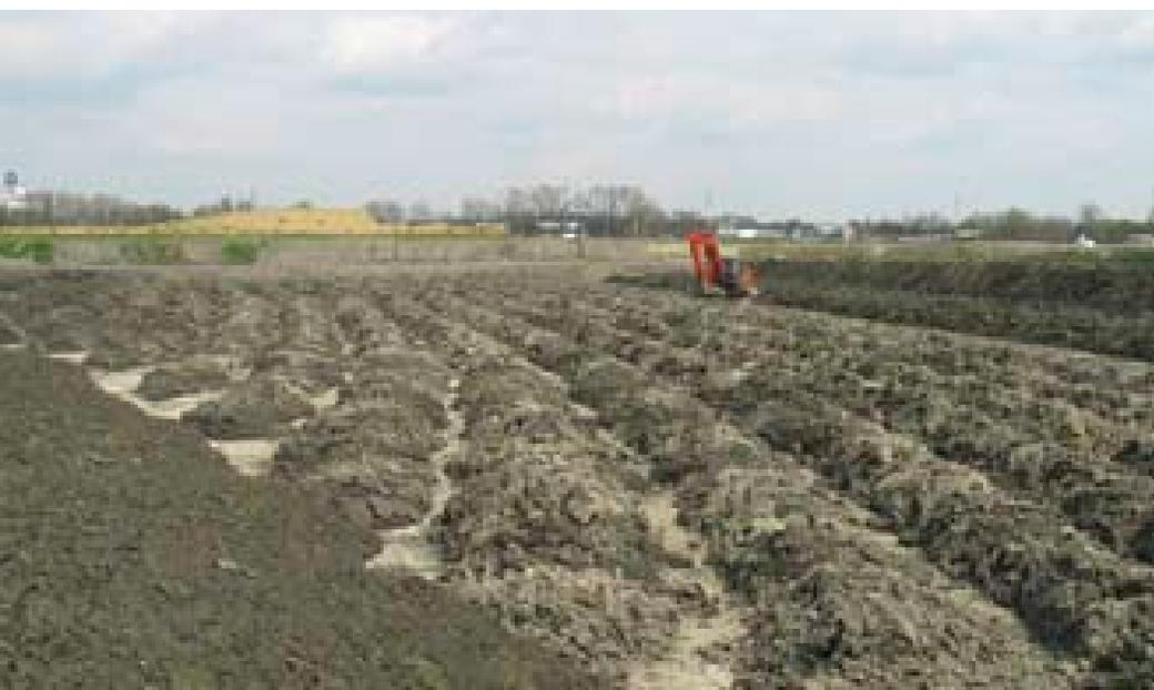
Figure 2. Dredged material being dried and worked upon at the Fasiver site. A total of 1.3 million tdm will be processed.
