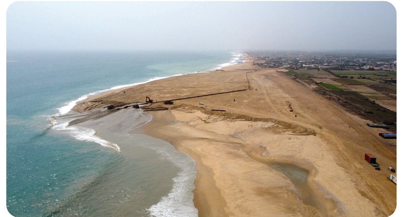
The sand motor under construction.
