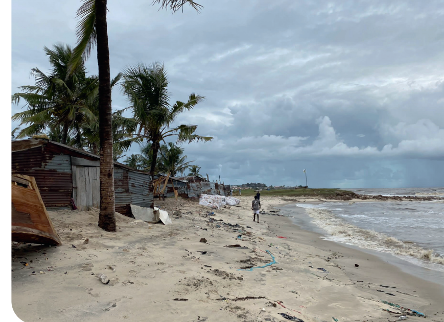
Coastal protection site in Beira, Mozambique, where Invest International and partners are working to safeguard the coast and 600,000 residents.
