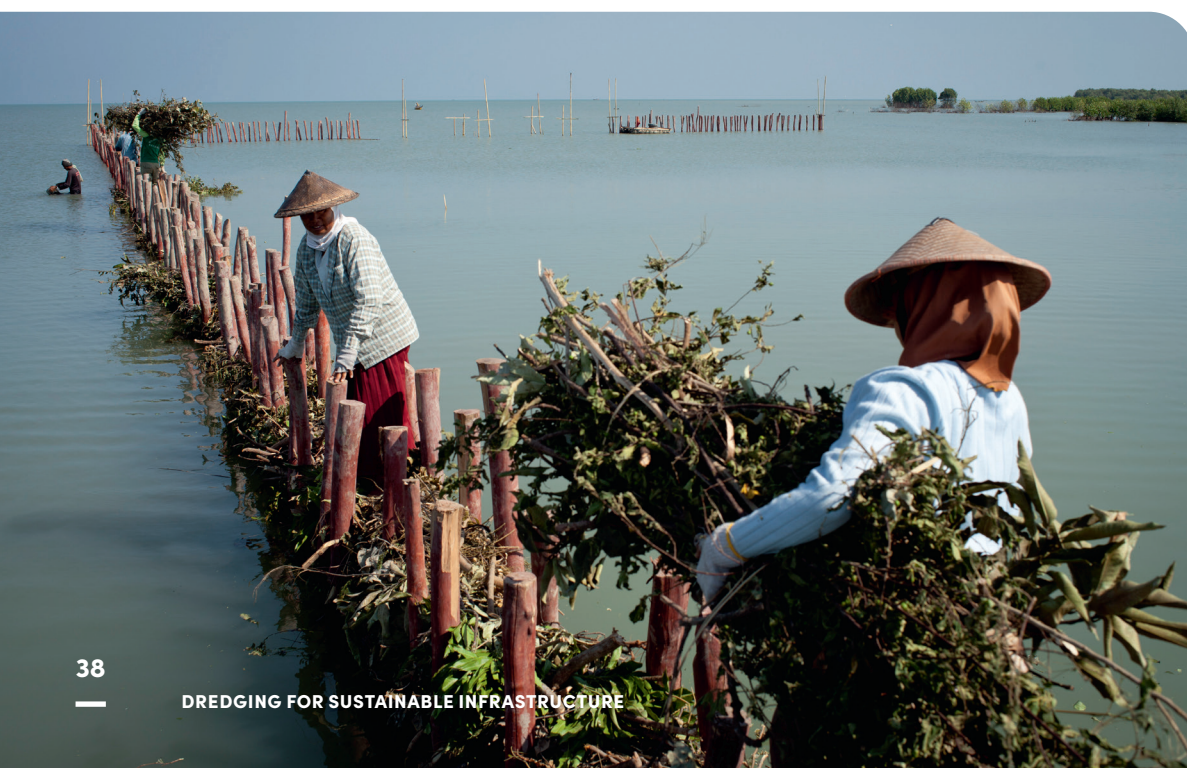
Trapping mud behind temporary permeable structures to stabilise the coastline and allow mangroves to seed and grow. @Wetlands International
